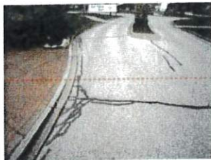
Crack-Seal - Example 1
