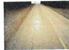
Crack-Block – Severe
