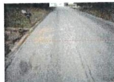
Crack-Block – Minor
