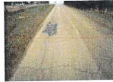
Crack-Block – Medium
