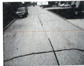
Crack-Seal - Example 2
